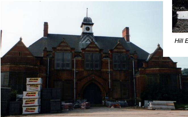
Administration block during demolition (Courtesy of Jim Whittamore)
